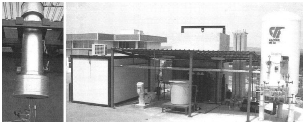
Figure 8. SCWO reactor and pilot demonstration plant of the High Pressure Process Group of the University of Valladolid (Spain).
